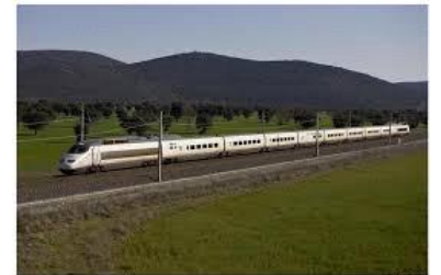
High Speed Train – station Puertollano
